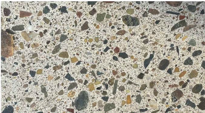
Existing exposed aggregate paving along Alexander Street.
